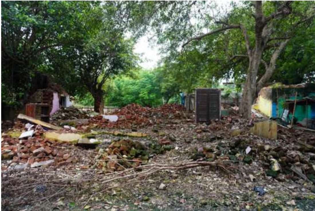
Figure 13: Construction near nesting site at Prabhavati Hospital, Gaya
