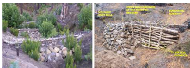
Source: Tardio et al (2017) Use of local raw material for check dam construction
